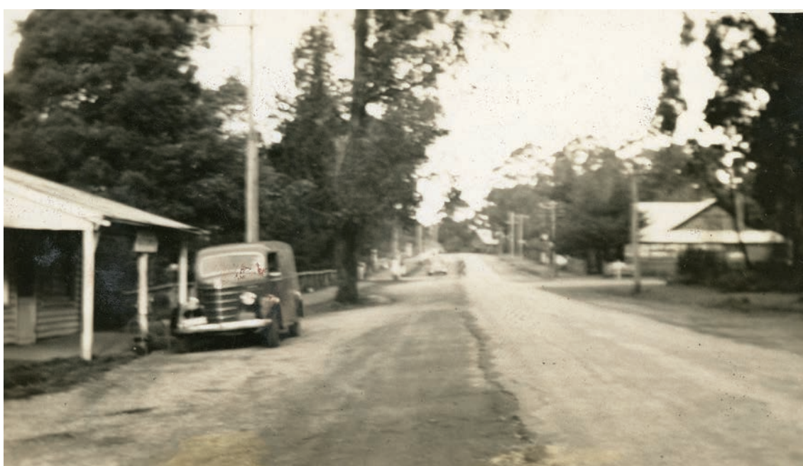
Les McAllister's delivery van parked outside the butcher shop in Monbulk's main street 1938. Emerald-Monbulk Road can be seen on the right.
